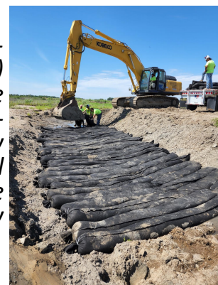
Biochar being installed into Elm Creek in the Tar Creek Superfund site 2022
